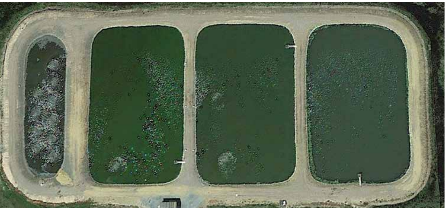
The Inkom wastewater treatment plant is an example of a small lagoon-based facility. / Google Earth
