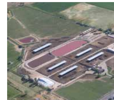
Dairy and waste water lagoons
