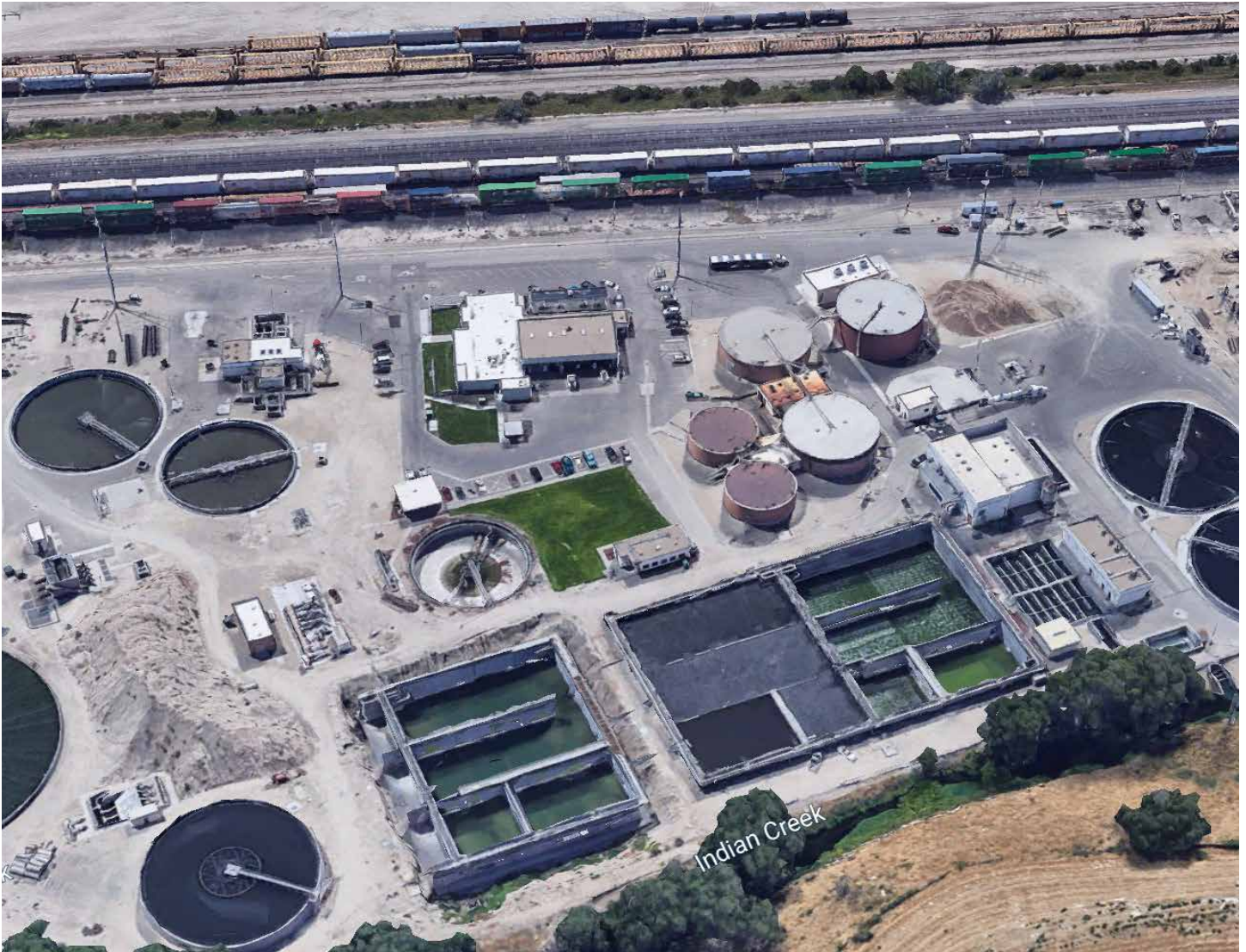
The Nampa wastewater treatment plant is an example of a large facility with mechanical and biological treatment. Google Earth photo.
